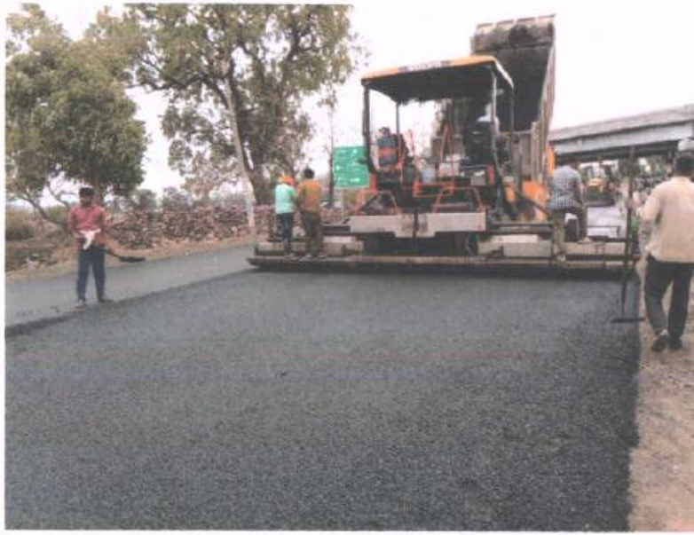
Km. 49+330 Laying work of Bituminous concrete at junction BHS
