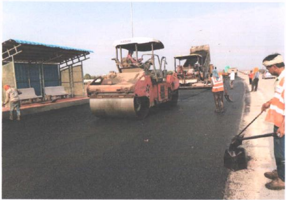
Km. 48+760 Laying work of Bituminous concrete at Bus bay LHS
